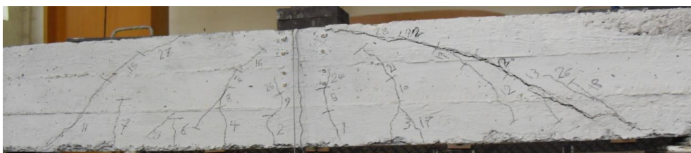
Figure 10: Crack Pattern for Specimen (B-A-3)
