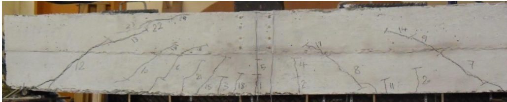
Figure 12: Crack Pattern for Specimen (B-C-3)
